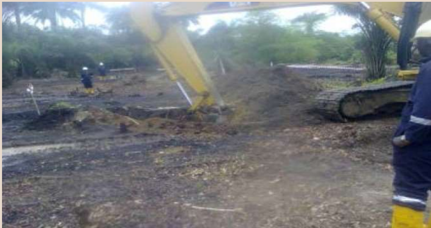
EXCAVATION AT POLLUTED SITE
